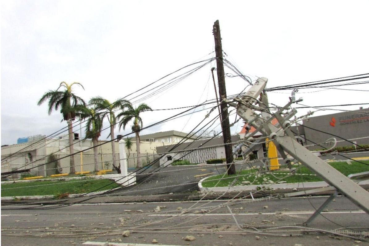
*Figure 23 - Fallen wooden and concrete electric distribution pole at Puerto Rico Highway 65*
